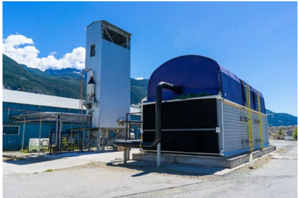
Carbon Engineering's pilot plant in Squamish, British Columbia
